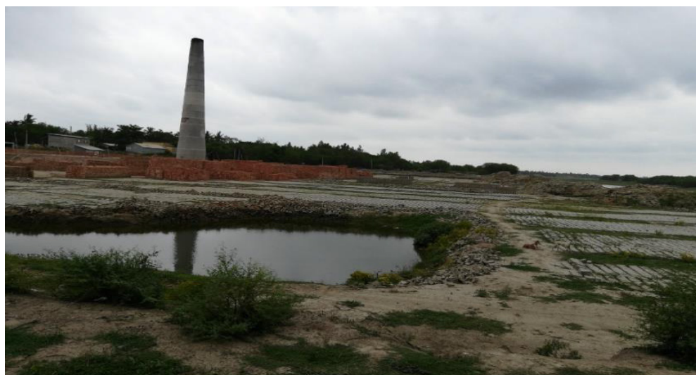
Figure 3.13: Brick Kilns alongside river Kaliaghai at ch. 42.70 km
