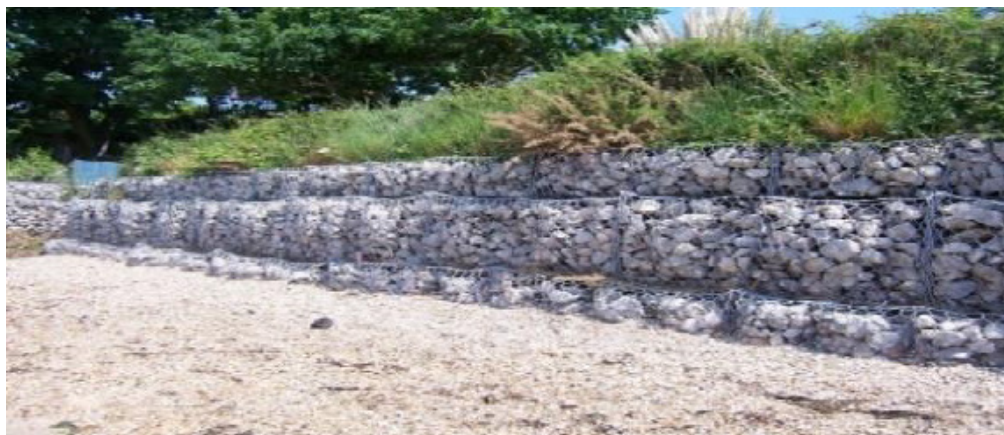
Figure 3.5 : Image of Boulder Pitching in sausage crate
