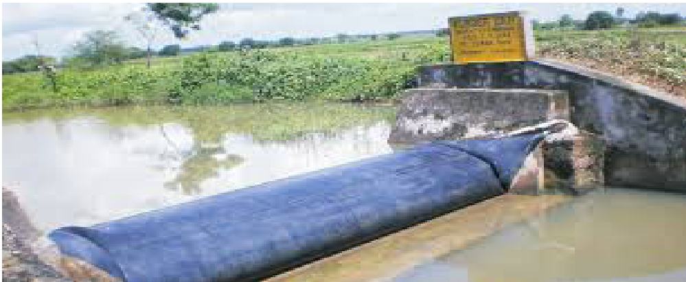
Figure 3.14: Image of a typical Rubber Dam
