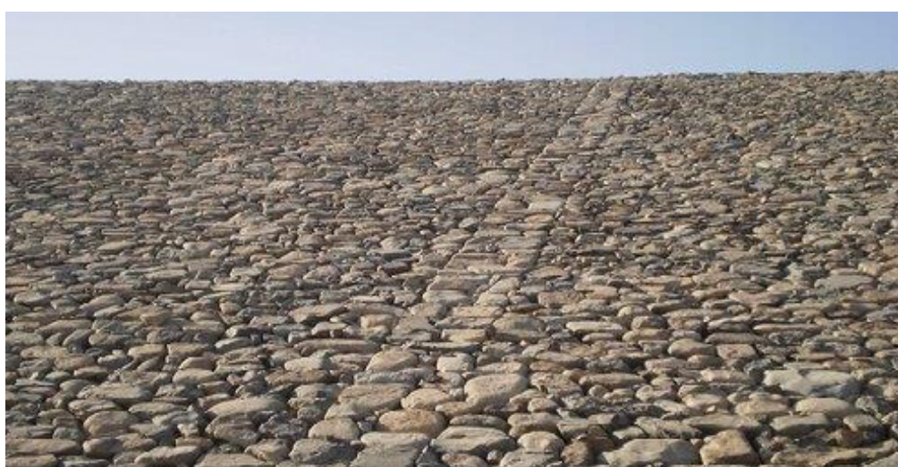
Figure 3.6 : Image of Loose Boulder Pitching
